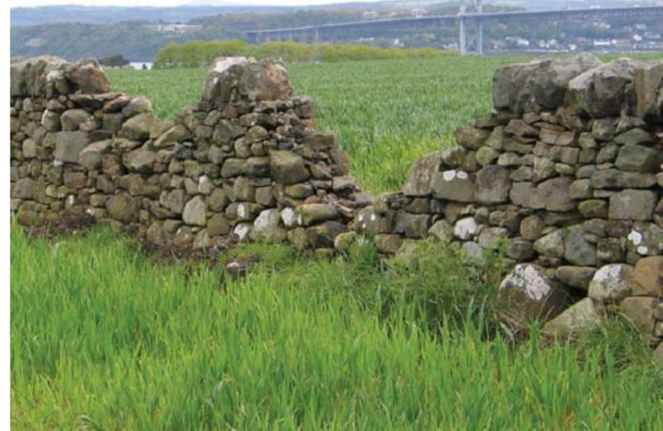
If there is inadequate drainage water may undermine the foundations of a wall leading to collapse. Flooding is a threat where there is a stream close to, or passing under a wall where an appropriately sized gap has not been built into the structure.
