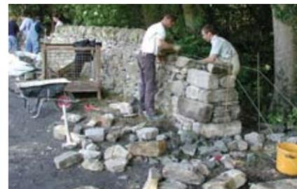
*Rebuilding a section of dry stone walling, note batter frame and wall head*
