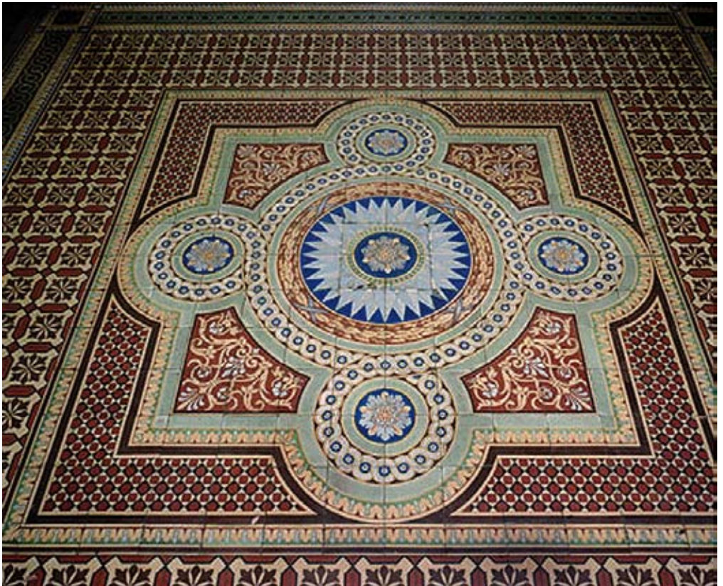
Polished encaustic tiles in a late 19th C hallway in Aberdeen . Scran 000-000-486-195-C
