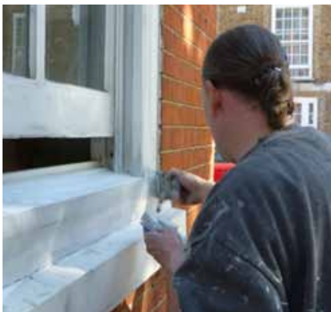
02/03 Before installing any draught-proofing to windows identify and make any repairs that are needed first. © English Heritage/Chris Wood/Robyn Pender
