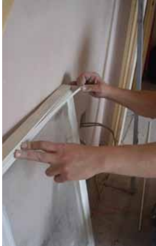
10 A brush pile seal being inserted into a window sash © Core sash windows
