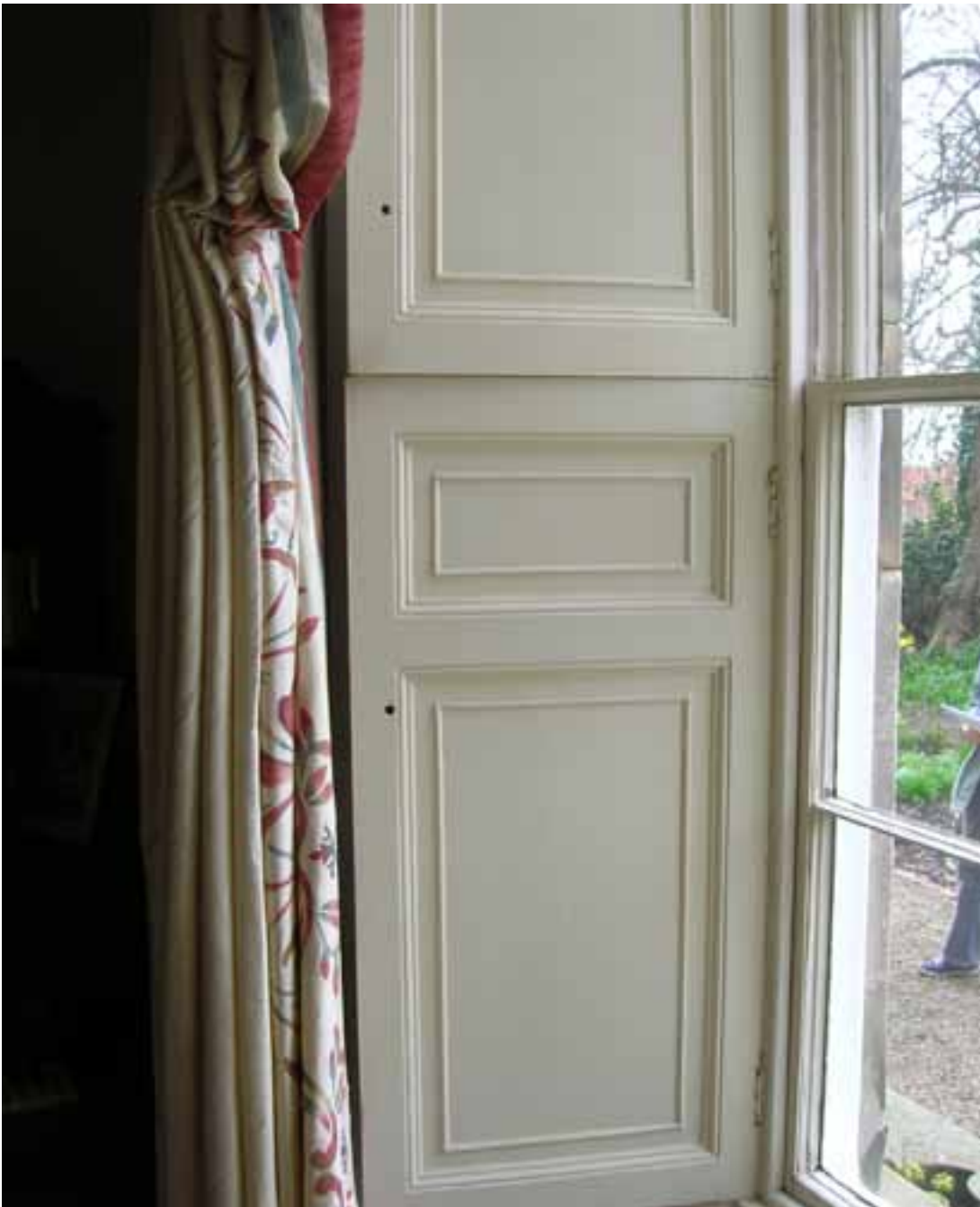
12 Shutters can be draught-stripped which will minimise heat loss when the shutters are closed at night © Linda Hall
