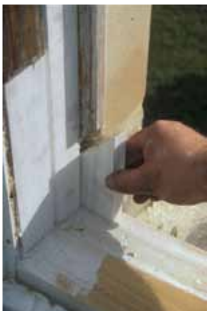
02/03 Before installing any draught-proofing to windows identify and make any repairs that are needed first. © English Heritage/Chris Wood/Robyn Pender
