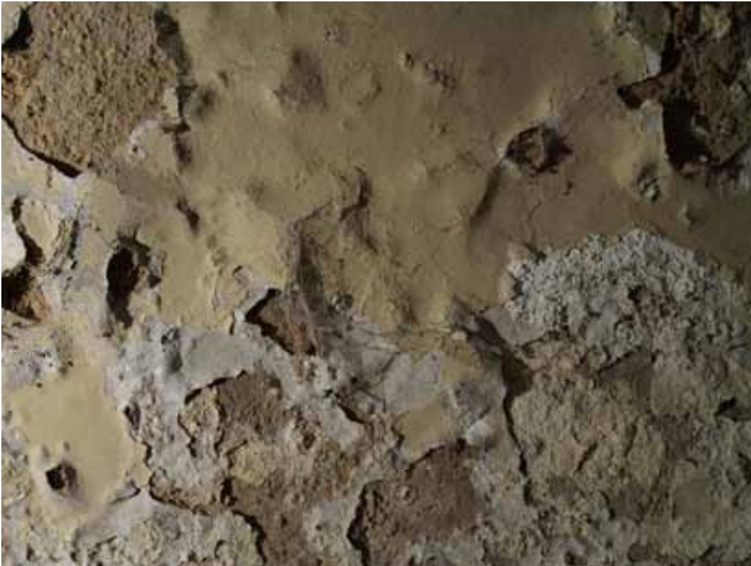
08 Many salts are hygroscopic and so exacerbate the problems of damp by attracting and holding moisture © Tobit Curteis Associates
