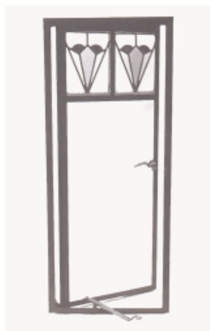
A typical steel window of the inter-war period
