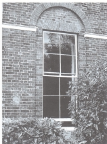
Cast iron sash window of c1805 in Essex
