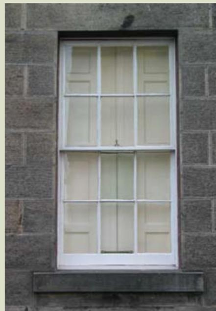
a latch attached to the shutters at meeting stiles, when they were closed it would be activated to hold the shutters in position.
