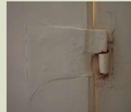
*Hinged connection between secondary and outer shutter leaves and outer shutter leaf and window jamb*
