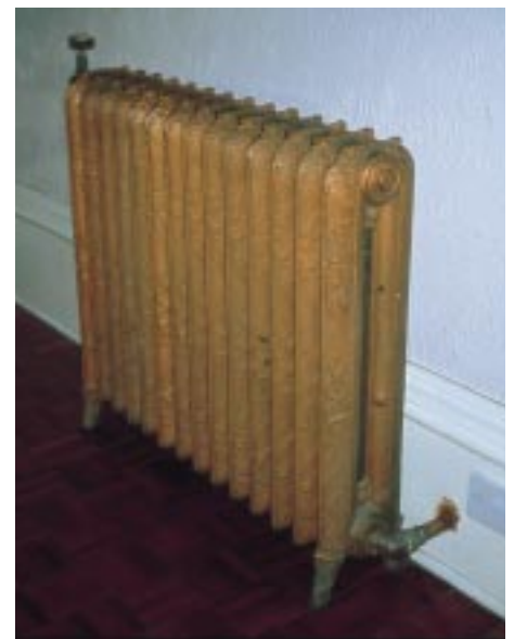
Figure 15 Examples of early cast iron stove and radiator which are still in use. Items such as these should continue to be used and if necessary refurbished to improve efficiency. (Photograph of stove courtesy of Robyn Pender; photograph of radiator by Chris Wood)
