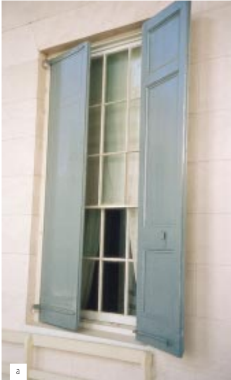
Figure 10 Shutters are not just historically important, they can provide significant thermal improvements as well as enhanced security and reduction of dust and noise. (Photograph: (b) courtesy of Matthew Slocombe and the Society for the Protection of Ancient Buildings; (a), (c), (d) and (e) by Chris Wood and other members of English Heritage Building Conservation and Research Team)
