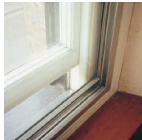
Figure 9 Secondary glazing can provide very effective thermal improvement. In historic buildings its successful insertion depends on fitting within the reveal in such a way as not to damage historic fabric. However, secondary glazing can sometimes produce an unsatisfactory reflection when viewed from the outside. (Photograph courtesy of Kit Wedd)
