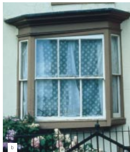
Figure 5 Historic glass, especially Crown glass, is rare and cannot be reproduced today. Where examples such as the middle right pane survive, they must be preserved. (Photograph courtesy of Treve Rosoman)
