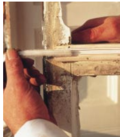
Figure 8 Draughtproofing strip being inserted into a routed channel on the bottom rail of the top sash. (Photograph courtesy of Ventrolla Ltd)
