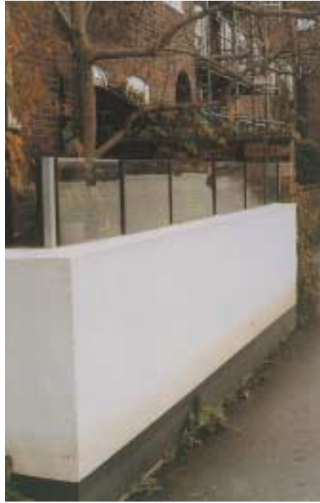
Figure 8 A boundary wall facing the River Thames in Hammersmith, West London, has been rendered to provide a flood barrier. Its height has been increased with a visually unobtrusive screen of toughened glass. (John Fidler)
