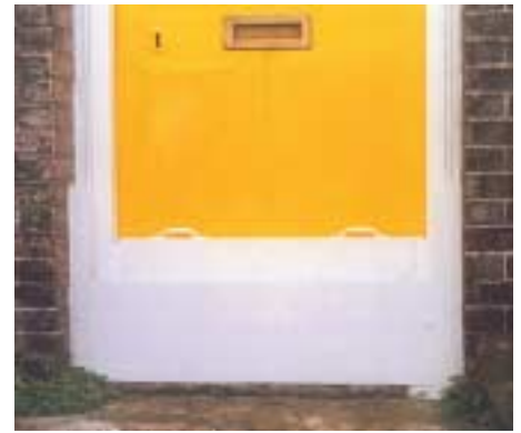
Figure 16 (above) Double layer barriers (see Fig 15) in position in front of an eighteenth-century door (John Fidler)
