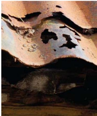
*Accelerated corrosion by overlaying sheets and causing capillary action*
