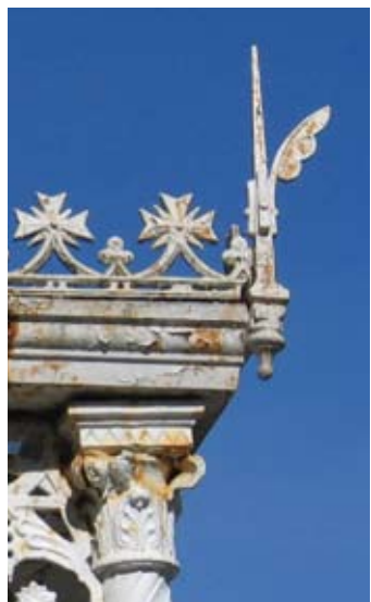
Cast iron finials can be fractured leading to the partial loss of decorative elements
