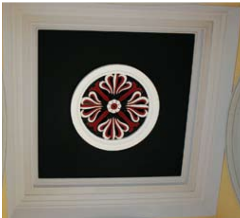
Closed up air vent in public building.
