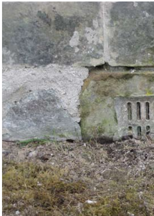
Despite recent masonry work to the elevation, this sub floor vent has
