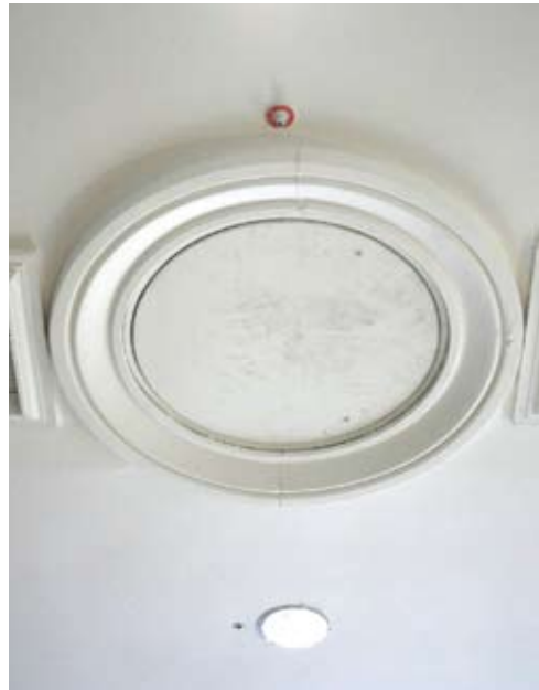
A decorative air vent at the top of 19th C stair.
