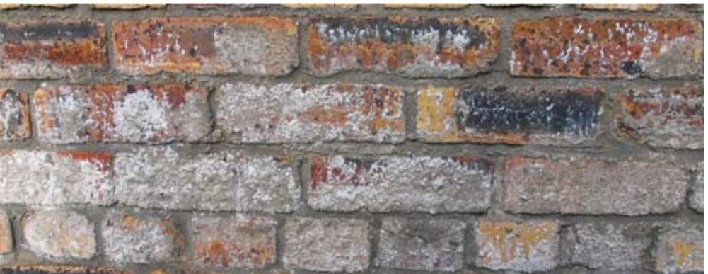
cases a thick build up of white crystals can form. This illustrates that salts are present in the construction and are migrating to the surface. The problem of efflorescence can be exacerbated by the improper use of cement mortars during repair. To prevent significant deposits of efflorescence from causing serious damage to bricks it needs to be regularly brushed off the surface using a bristle brush and the source of water causing the build up of the deposits to be stopped.
