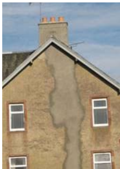
A flue relined from the outside.
