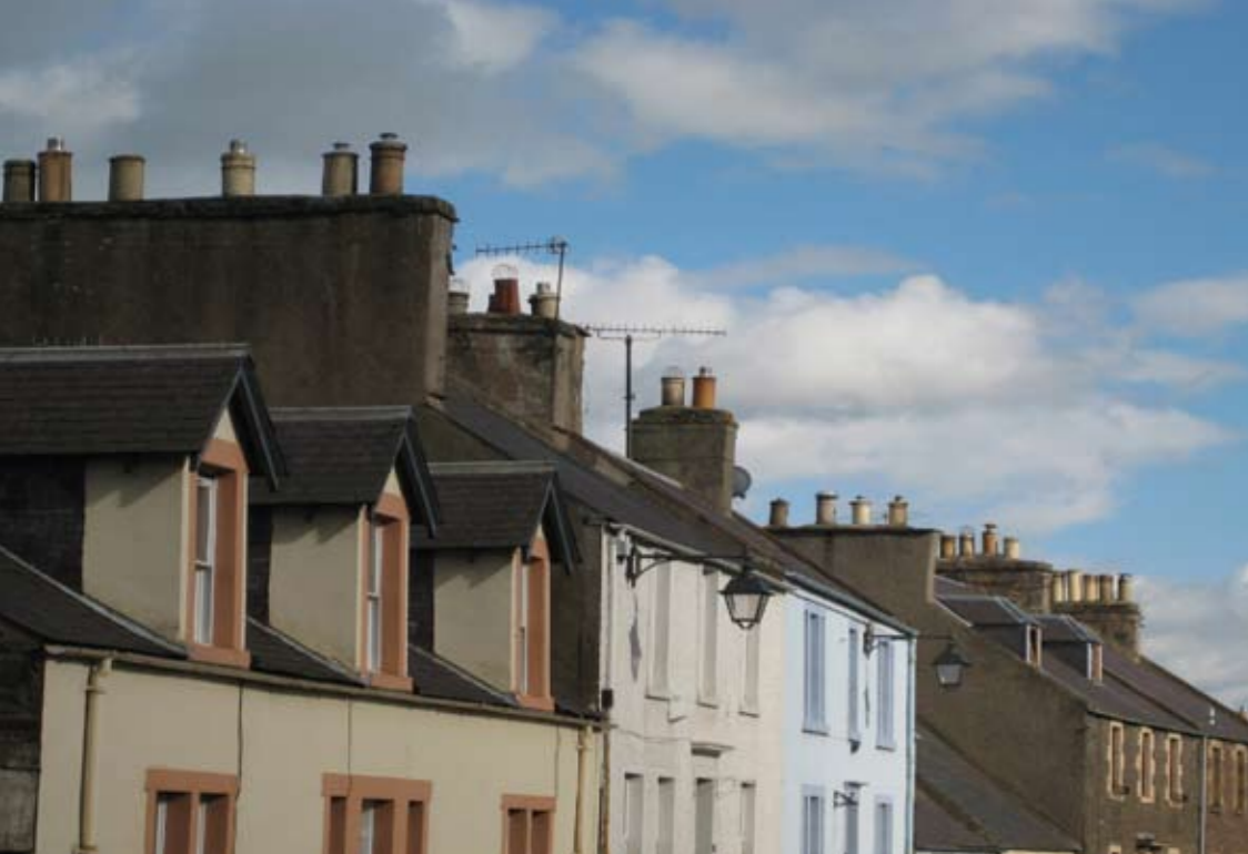
Chimneys and cans are a dominant and distinctive feature of the urban environment.
