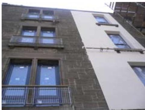
*Fig 11. External insulation applied to an unlisted tenement has dramatically changed its architectural character.*
