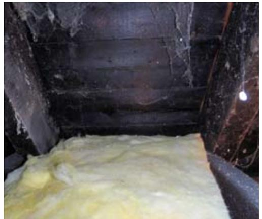
*Fig 3. Mineral wool insulation can also be laid between rafters and joists, but with care not to inhibit air movement.*
