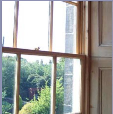
*Fig 10. Existing sashes re-glazed with DG units.*
