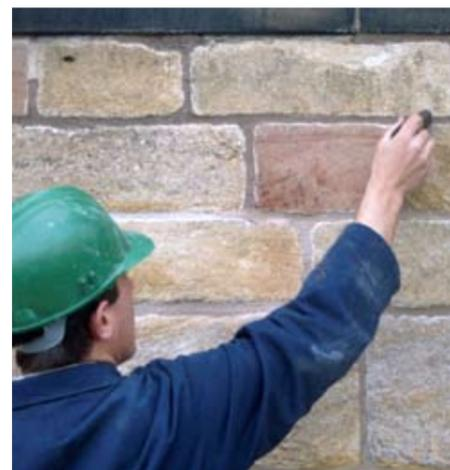
Mortar may be inserted into the joint from a board held adjacent to the wall face by using the side of a thin steel blade or similar tool. If the joint width allows, regularly inserting a thin wooden (or other material) spatula into the joint to compress the mortar as work progresses will help ensure that the joint is properly filled.
