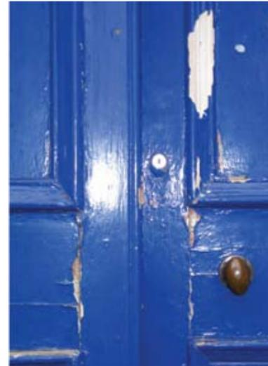
*If not regularly maintained paint will begin to peel from doors leaving them vulnerable to further deterioration.*
