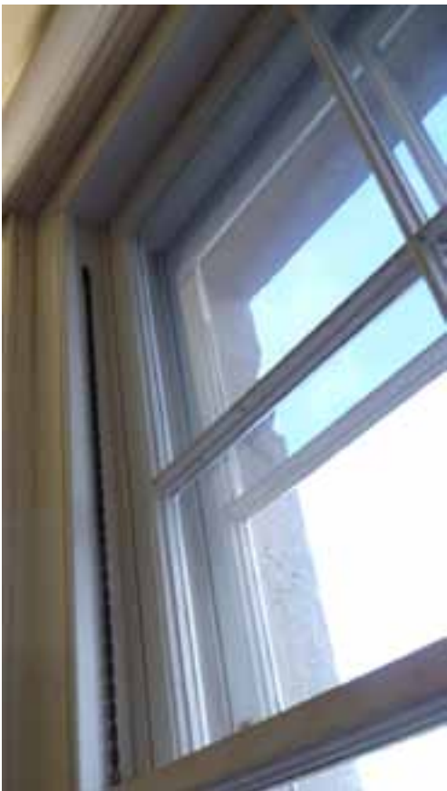
01 A 19th century secondary glazing arrangement comprising two sets of double hung sashes © English Heritage/David Pickles
