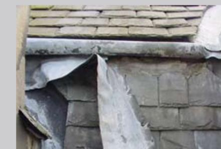
This should consider the overall condition of the lead, how long it has been in place, whether there are any inherent design faults, and whether or not there is any interaction occurring between other nearby materials or growths.
