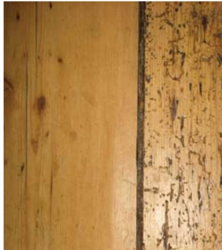
*19th C flooring, showing wood beetle attack (no longer active) on the softer timber.*
